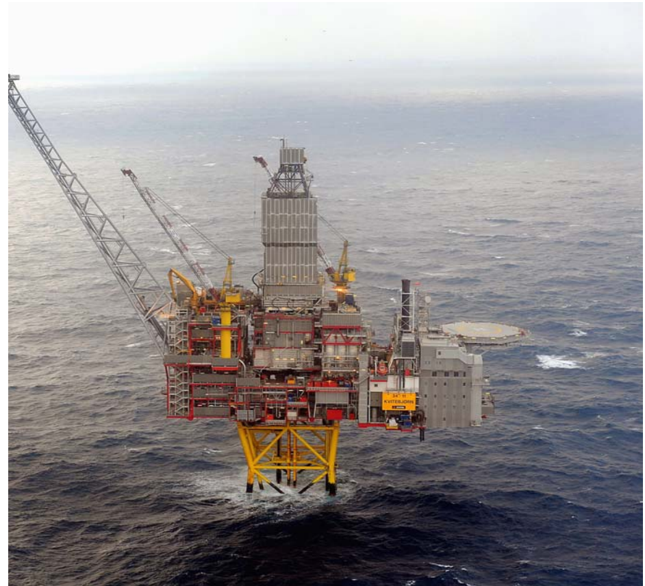
Unique Kvitebjørn pipeline repair
